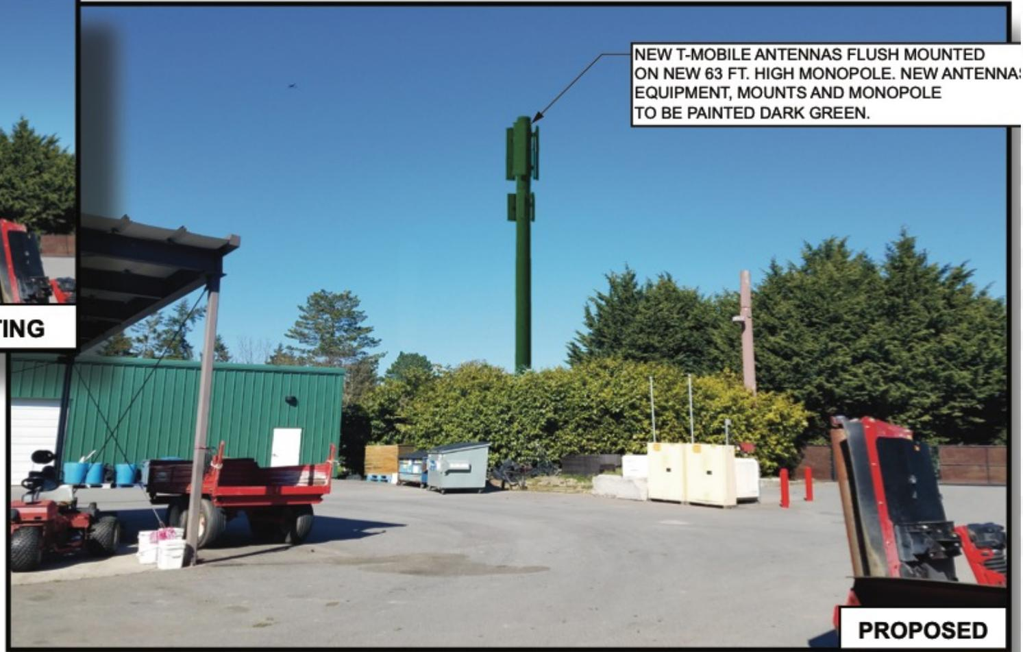
NEW T-MOBILE ANTENNAS FLUSH MOUNTED ON NEW 63 FT. HIGH MONOPOLE. NEW ANTENNA EQUIPMENT, MOUNTS AND MONOPOLE TO BE PAINTED DARK GREEN.
