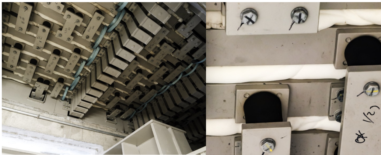
Figure 4-4. Underside of the MEJ with viscoelastic foam strips stuffed into the gaps.
